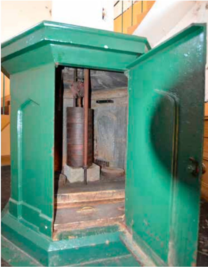
TOP LEFT: The eleven circular weights each of 22 kg rest at the bottom of the 22 ft (6.7 m) winding shaft. TOP RIGHT: The stone staircase leading to the first floor.
